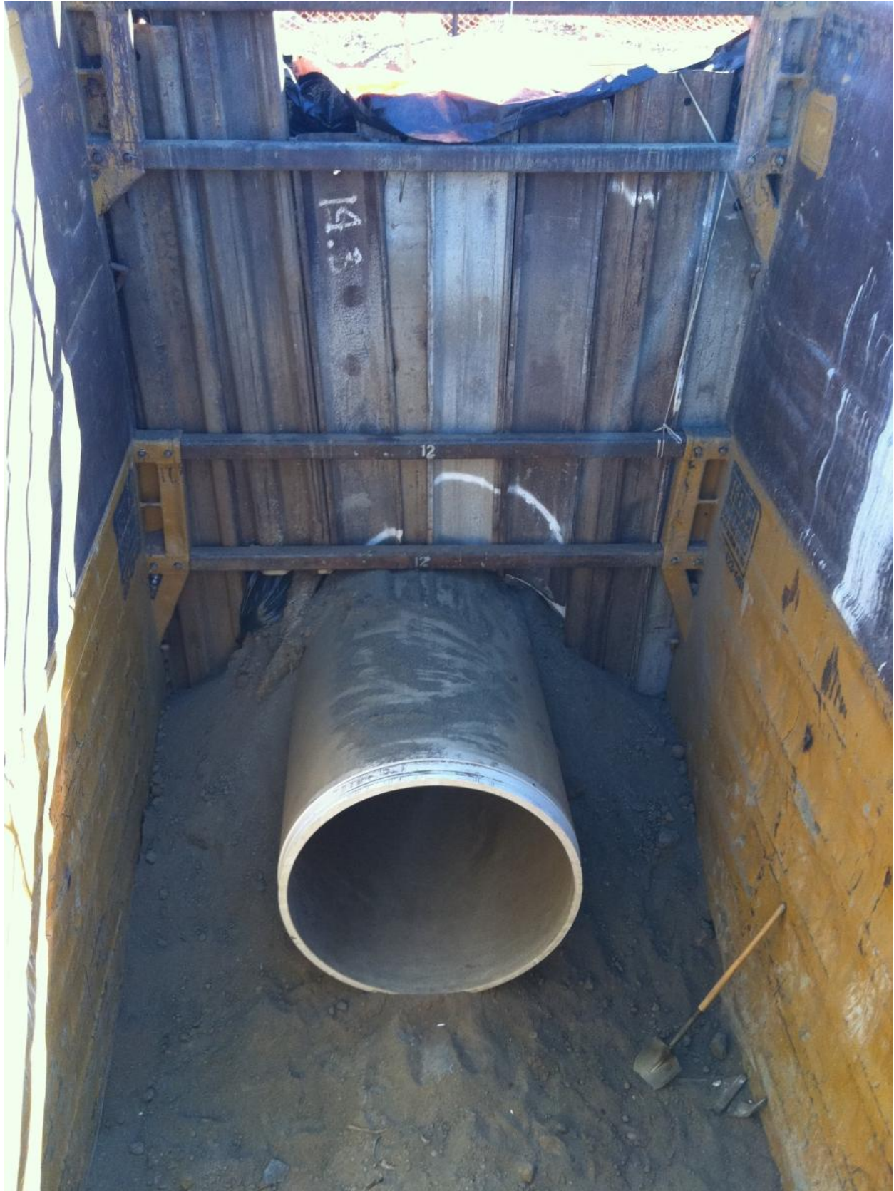
Receiving bore pit showing completed bore. Photo courtesy of Jeff Smith.
