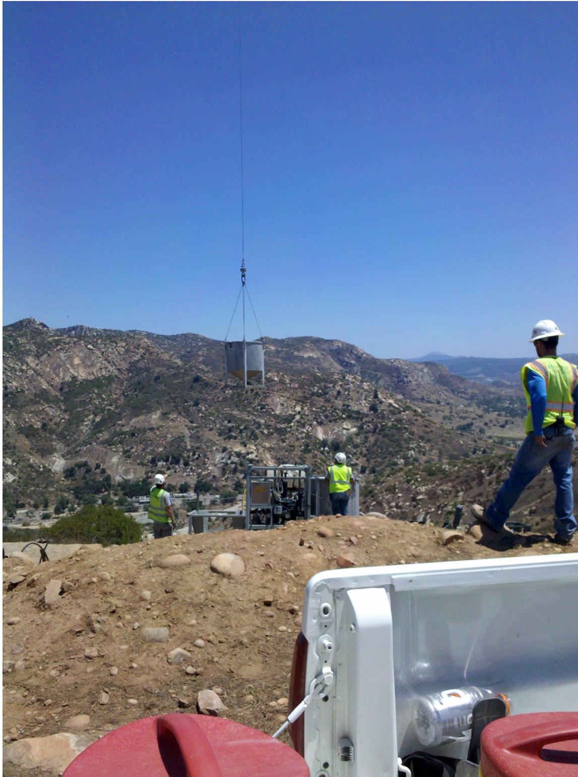
Micropile grouting at CP42-1. Photo courtesy of Rosina Gallego.
